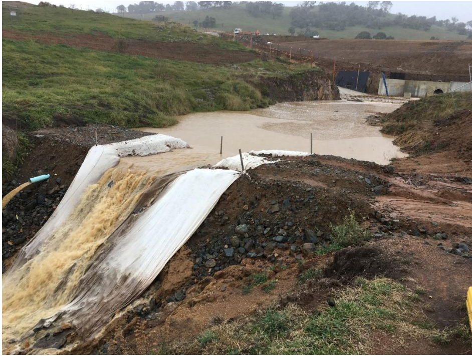
Figure 17. Deep Creek sediment detention pond illustrating the failure of the pond to trap fine sediments, June 2020. Source: ACT Waterwatch.
