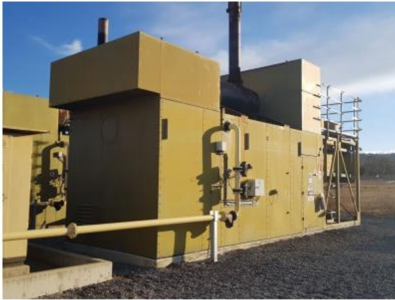
Landfill gas fuelled power generation units at the Mugga Lane Resource Management Centre. Source Energy Developments
